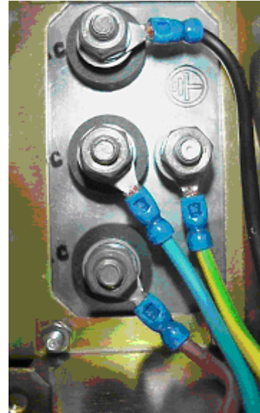
Figure 3-3: AC Input Terminals
